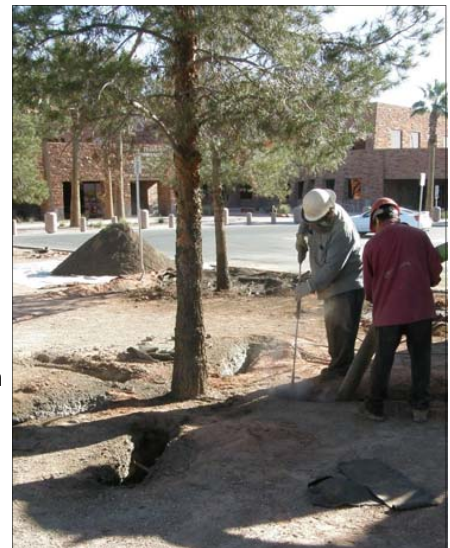
After creating radial trenches, soil is replaced with rich organic material.
