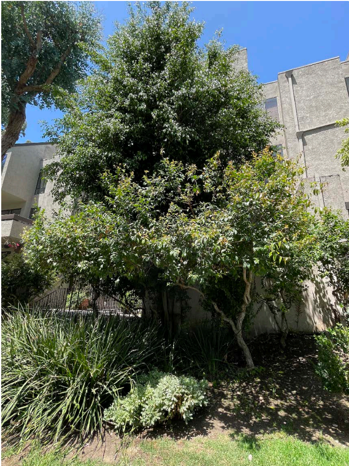
PHOTO - Ficus benjamina - This tree is near a foundation wall. Exploratory trenching should be performed on back of tree, near wall, and roots examined and possibly root pruned, and a root barrier installed to reduce impact from the massive Ficus roots.
